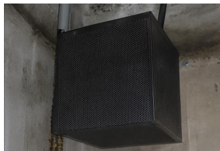
Fig. 1: Trap/screening baskets at the outlet of the aeration basin to prevent carrier washout
