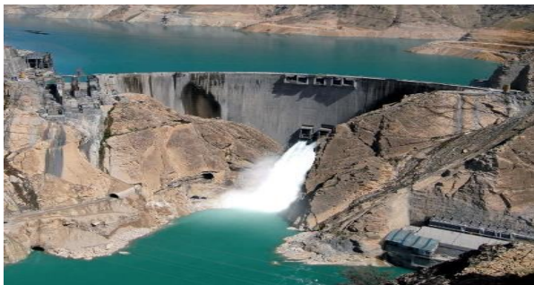
Fig. 5: A view of the arched concrete dam of Karun 4
