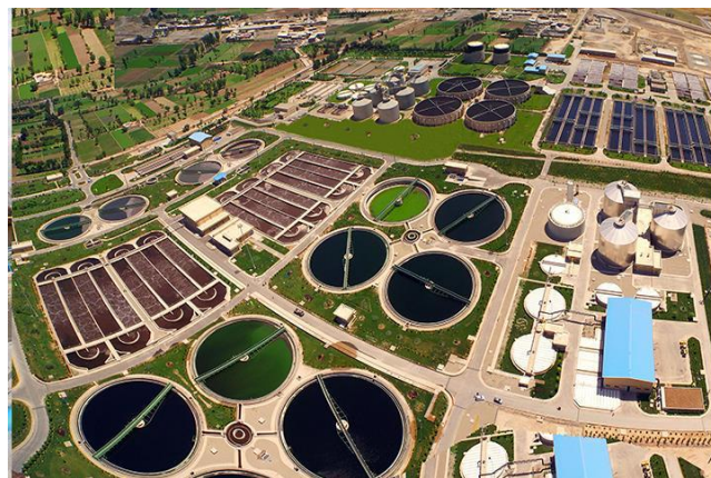
Fig. 3: South Tehran sewage treatment plant
