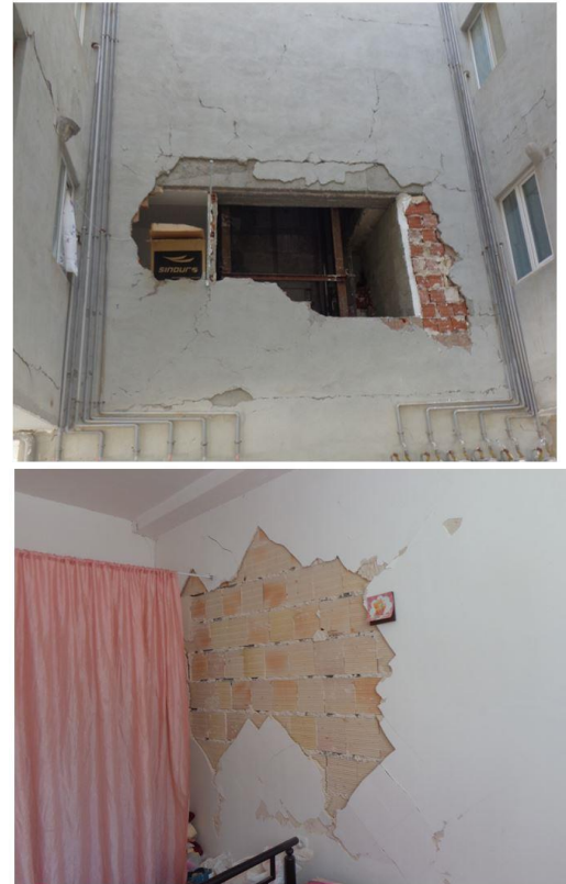
Fig. 1: Non-structural members damage in the Bojnord 2017 earthquake. The pictures were taken by the engineers of the Mandegar Structures Q.C. & Inspection Company.
