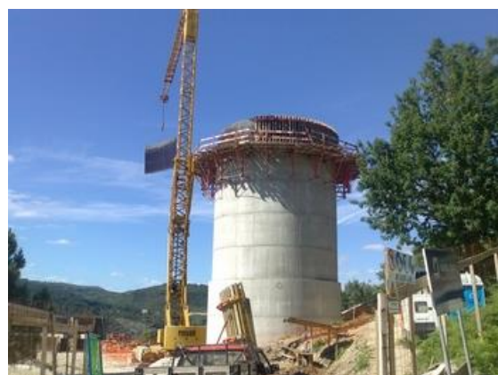
Fig. 1: Construction steps of a surge tank
