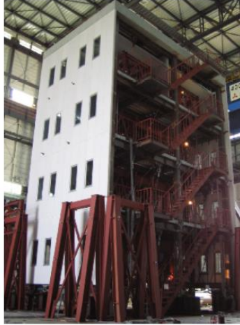
Fig. 3: Full-scale 4-story steel structure after the completion of the NIED shaking table [42].
