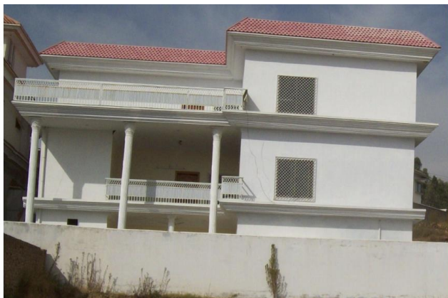
Three Storey Unreinforced Brick Masonry Building
