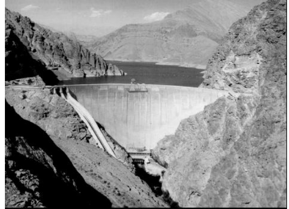
Fig .5: Downstream view of Amir Kabir arch dam
