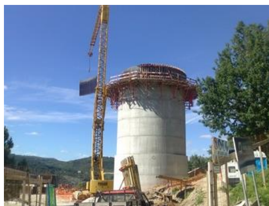
Fig. 1: Construction steps of a surge tank
